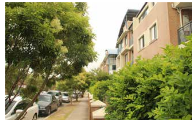
7-19 James Street frontage
