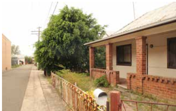
No. 9 Raphael Street looking south
